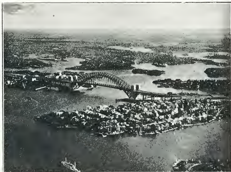
THE HARBOUR BRIDGE
