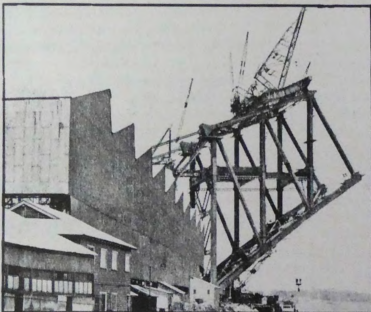
Fig. 6. Commencement of Arch Erection, showing Straining Cables and Raking Struts
