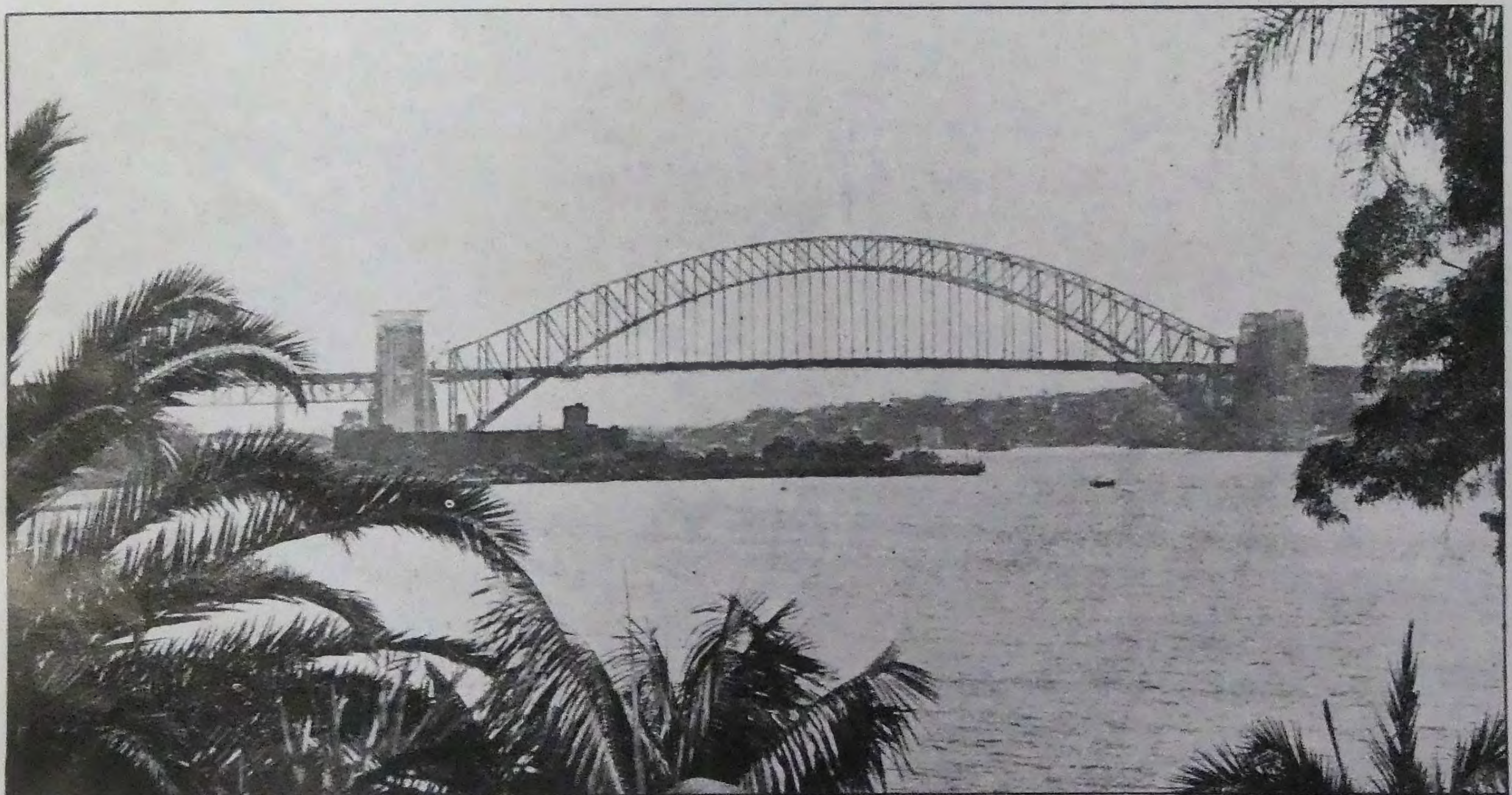
Fig. 1. The Main Arch of the Sydney Harbor Bridge
